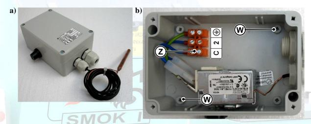
Fig. 14. a) STB temperature limiter, b) STB with cover removed
